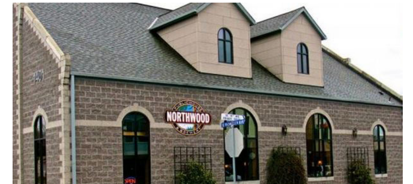
The Northwood is a brew pub in Battleground Village with a pub on the ground floor and brewery production above.
